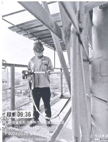
矿渣微粉1#成品仓废气排气筒出口
