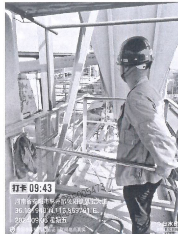
矿渣微粉2#成品仓废气排气筒出口
